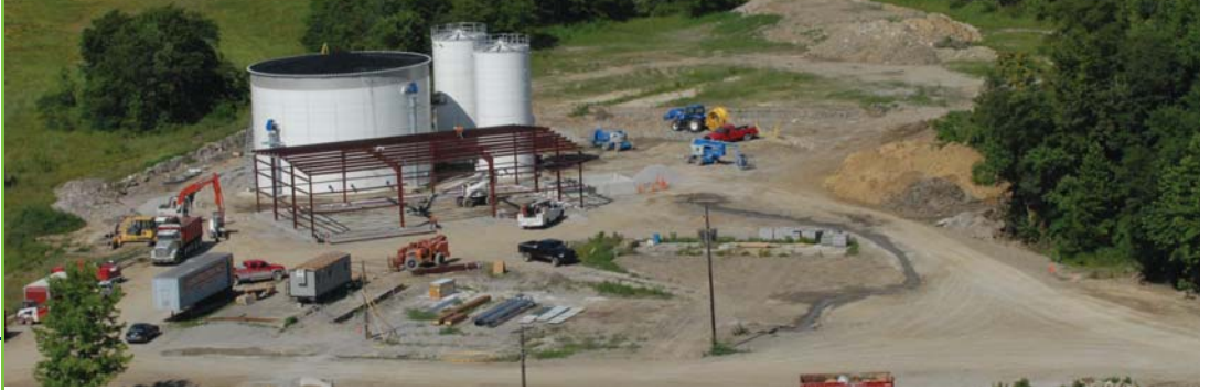
quasar's F825 system under construction in Zanesville, Ohio
